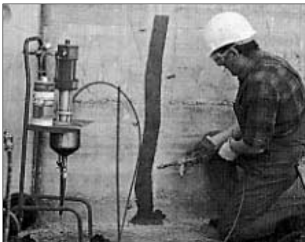
Figure 3.18: Injection de fissures
