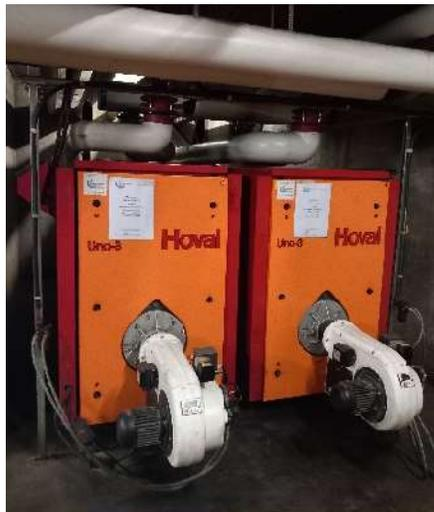
Figure 2 : Chaudières mazout – 2x 280 kW
