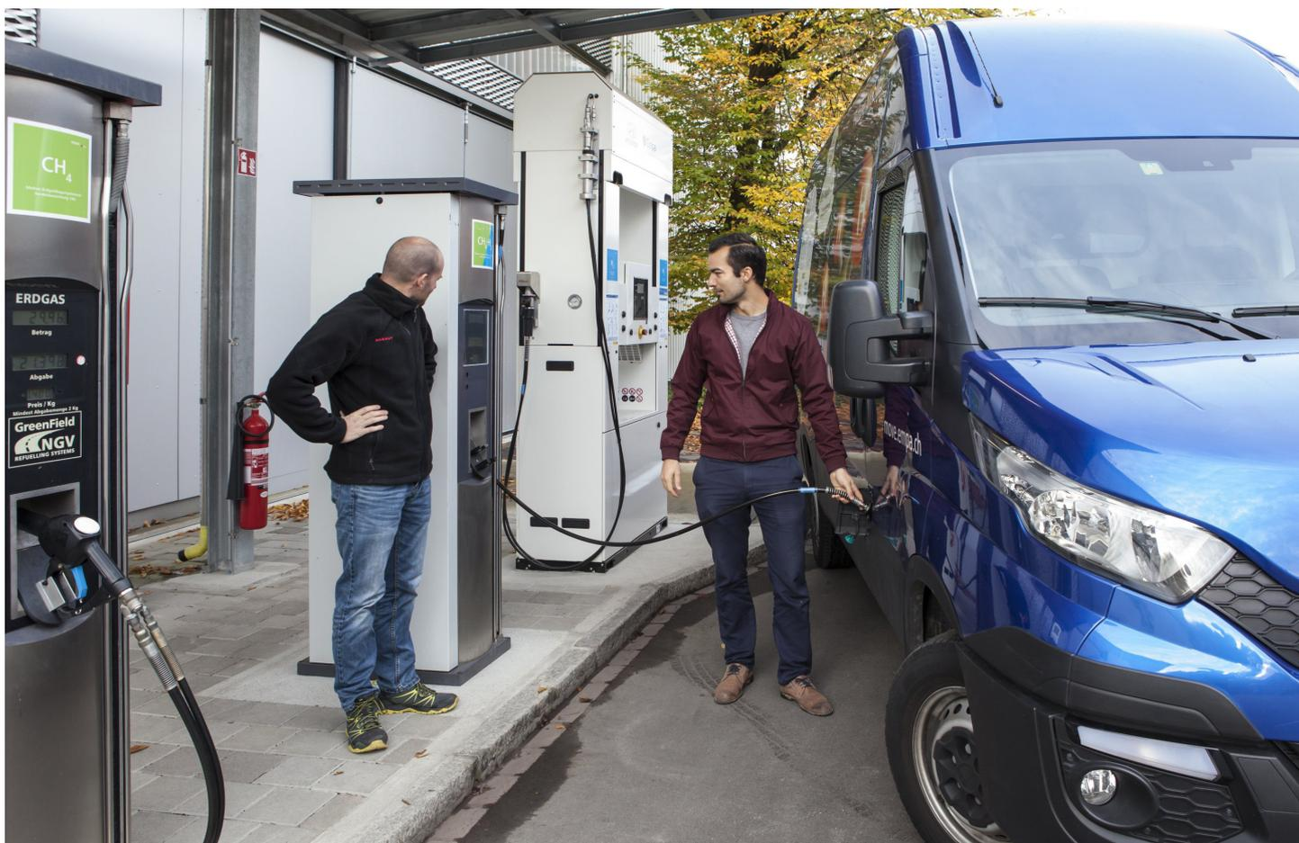
The three fuel dispensers of the “move” project at Empa provide different fuels: methane (front), a methane-hydrogen mixture (middle) and hydrogen (rear). Photo: Empa
