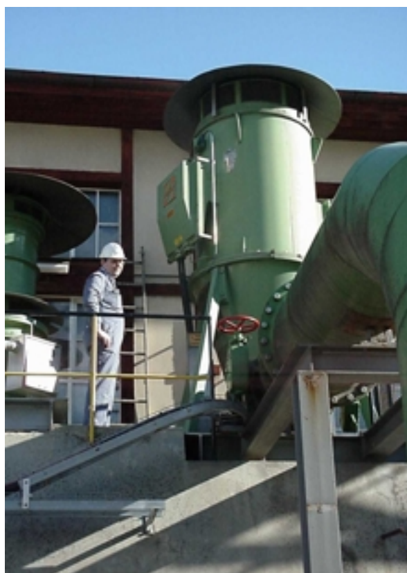
Figure 7: HS network water pump at Lonza (Source: Lonza AG, Visp)
