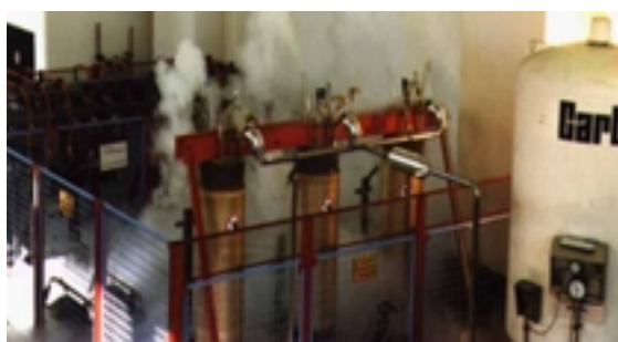
Figure 1: Prototype of a current limiter in a Swiss power plant (Source: ABB Research Centre)
