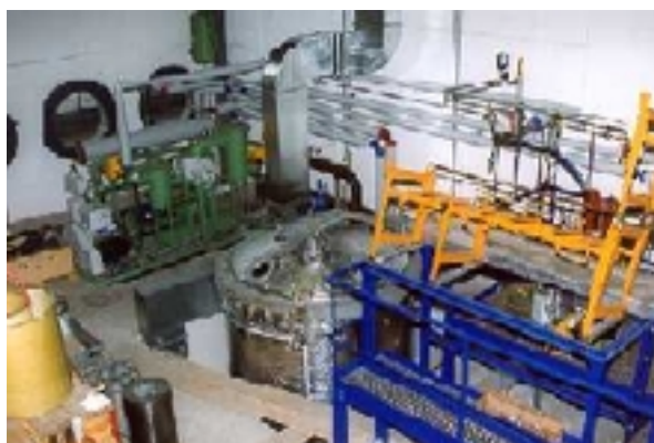
Production hall for high-temperature superconductivity transformer
