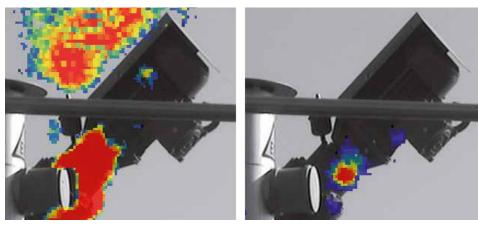
Gas losses at the agitator of a biogas plant. The areas in red represent high methane concentrations, while areas in blue indicate low concentrations. Left: before lubrication; right: after lubrication.
