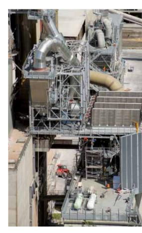
Waste heat from a cement factory can be used for producing electricity with the aid of an ORC (Organic Rankine Cycle) system.
