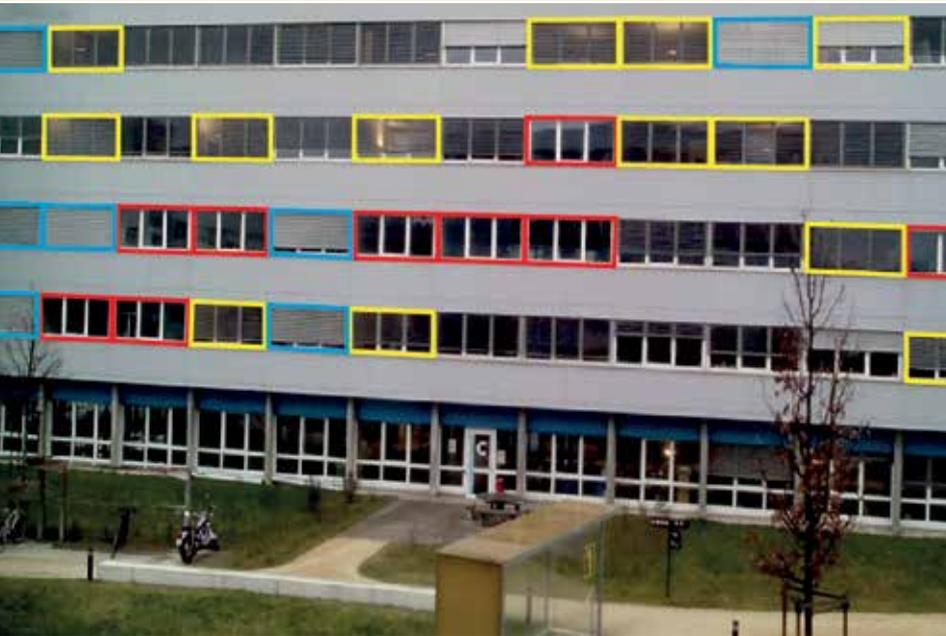
*West facade of an office building with manually operated blinds on a cloudy day: use of blinds is random and only a few are in the appropriate position (shown in red). The lights are on in some of the offices with the blinds partially drawn (shown in yellow).*
