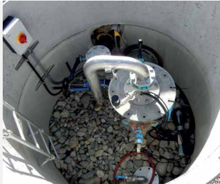
A near surface aquifer can be used as a geothermal heat source in Davos (left). View of the head of the 400 m-deep well (right) (image source: Municipality of Davos).
