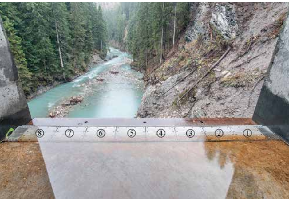
Geophone plate series at the outflow of the diversion tunnel at Solis: Metal plates, equipped with acoustic sensors which detect vibrations from impacting particles, serve to quantify the transport of solid materials (image source: ETH Zurich).
