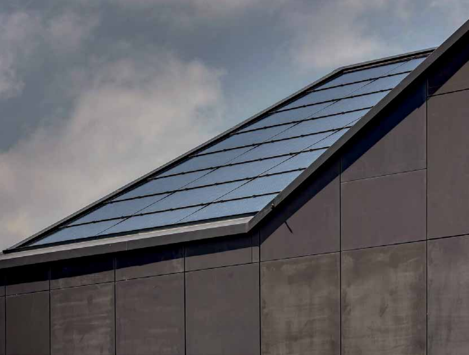
Integrated solar system in the energy self-sufficient house in Brütten (Source: Schweizer Solarpreis 2016, www.solaragentur.ch ).
