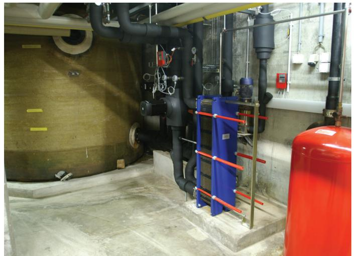
The heat exchanger (blue) absorbs the heat from the solar circuit and supplies it to the groundwater, which is stored in the groundwater tank (brown). Photo: B. Vogel
