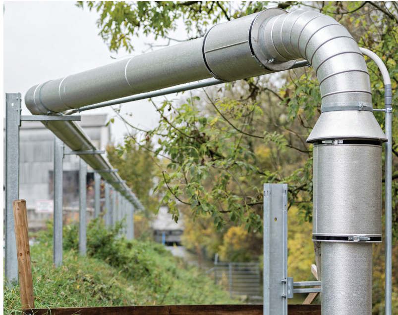
This 400 m long pipe is located in the industrial area of Weinfelden (TG) and delivers Meyerhans Mills' starch product to the adjacent paper mill of Model AG. Photo: Meyerhans
