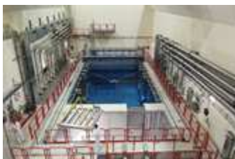
Fuel elements are also kept in interim storage at nuclear power plants (photo: underwater storage facility at Gösgen nuclear power plant). Source: Nuclear power plant Gösgen
