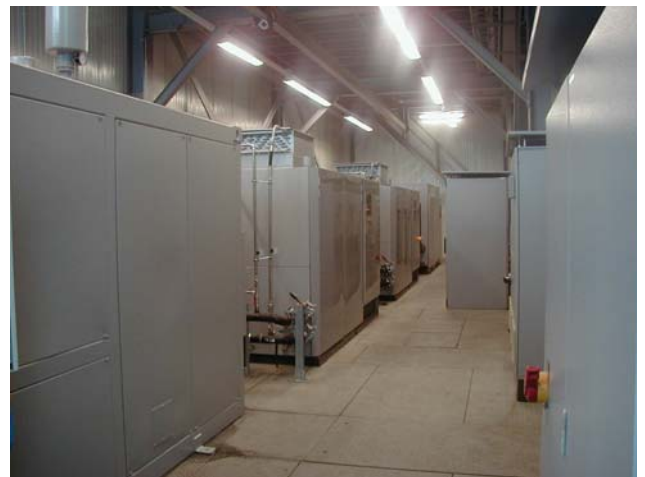
Fig. 2: Compressed air system
