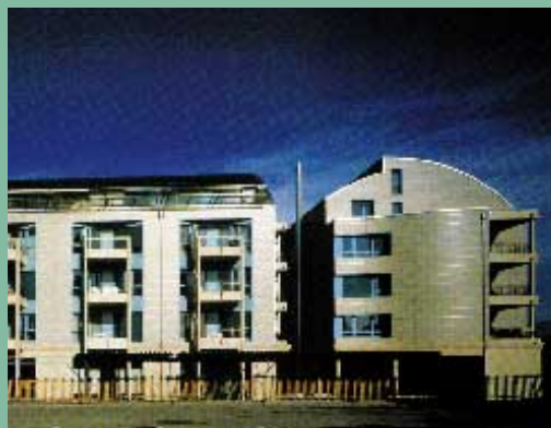
This apartment complex in Plan-des Ouates served as a demonstration project. By applying latest know-how, its energy index was brought down to 250 megajoules per m 2 – one third less than ordinary, comparable buildings.
