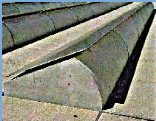
PV supports for flat roofs as an example of implementation: concrete bases each accommodate one PV module 120 cm in length and 52 cm wide. The weight of these bases alone is sufficient to ensure their ability to withstand strong winds.
