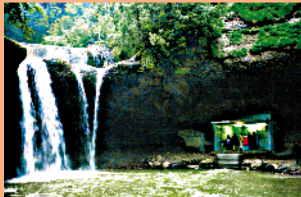
110-kW small-scale hydro on the Gonzenbach, Toggenburg, reactivated in 1996 with added environmental protection measures: original dam of 1894 (top left) retained, water duct underground, powerhouse (right) fitted with soundproof glass.
