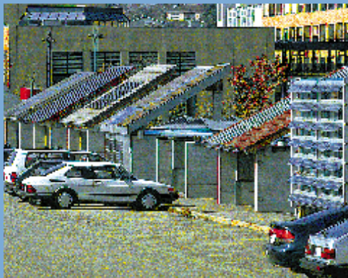
International co-operation in photovoltaics : PV systems operating in an IEA project at the Swiss Federal Institute of Technology Lausanne demonstrate their integration into buildings.
