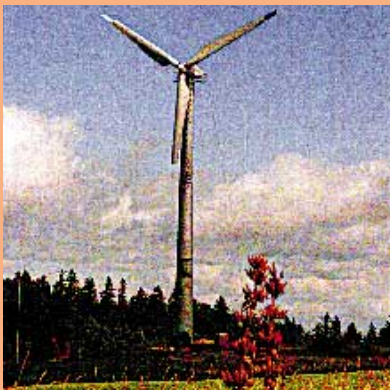
Obergrenchenberg 150-kW wind power plant (height 30 m, rotor diameter 24 m, 140'000 kWh/year): demonstration of performance, assessment of visual impact on the landscape.
