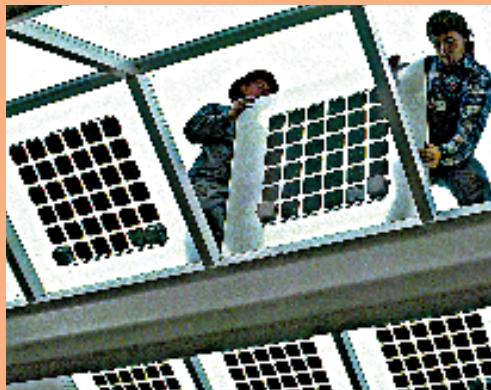
Transparent roof tiles which have been fitted with solar cells permit the integration of photovoltaic solar cells into buildings with simultaneous daylighting.
