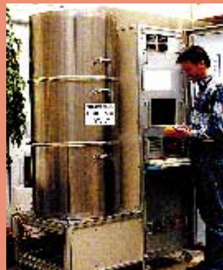
A 7-kW HEXIS system: in the casing cell stack and auxiliary equipment, on the right the electronic control unit.
