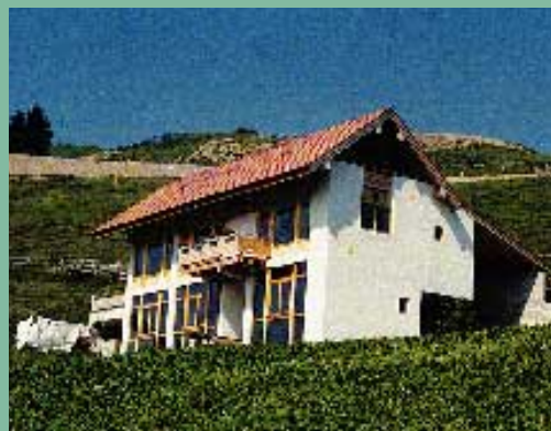
Traditional architecture can incorporate modern, energy-saving construction elements – this home at Gonten takes heat from air collectors and stores it in concrete ceilings integrated into the building shell.
