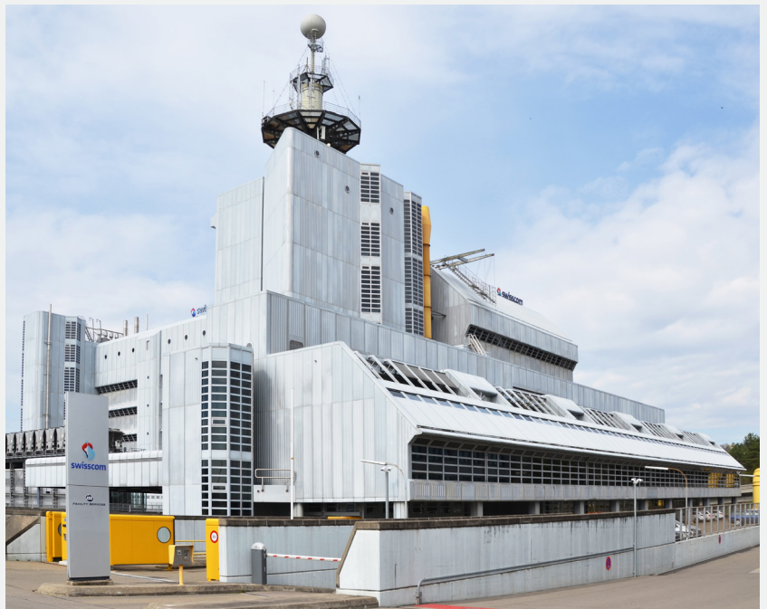
The CEST-DC study examined various sustainability aspects of data centers. Pictured: Swisscom's data center in Zurich-Herdern, which has been supplying heat to a regional heating network since 2012. Photo: Shutterstock
