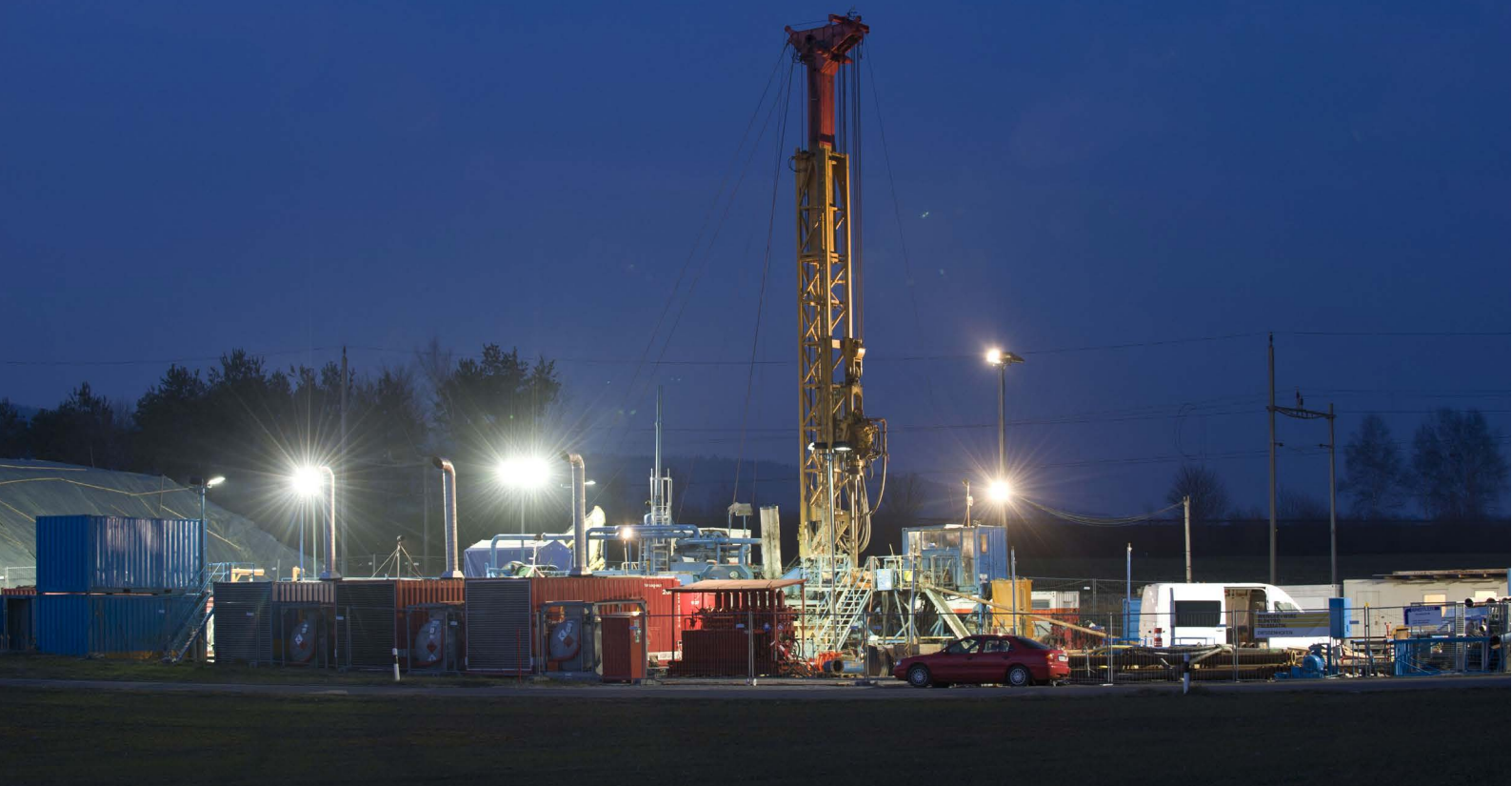
The drilling site for the first borehole (SLA-1) next to Grob Gemüse AG in the municipality of Schlattingen, Canton of Thurgau (source: Nagra).
