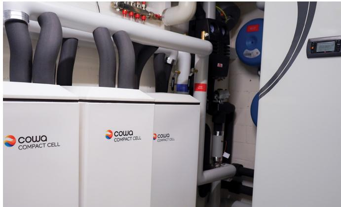
In 2023, Cowa Thermal Solutions introduced its first hot water storage tank based on phase change material with a melting point of 48 °C (pictured, three storage tanks connected in a cascade). The phase change material is based on sodium acetate trihydrate, a salt with a faint vinegar smell. In the PCM storage tank tested at HSLU, the phase change material is placed in a converted basement room or in an underground water tank. Photo: Cowa
