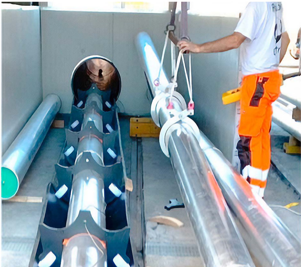
A roll system developed in-house is used for installation. The cable tubes are pulled into the protective tube using a pull rope (source: Hivoduct).
