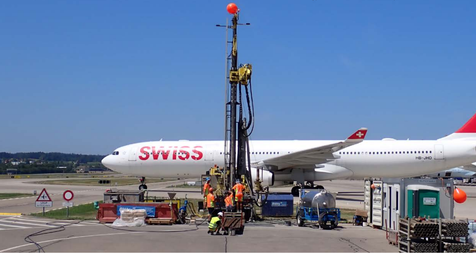
The first exploratory drilling at Zurich Airport site was carried out in 2023. It confirmed the presence of water-bearing gravel layers at the base of the glacial channel (source: Geo Explorers AG).
