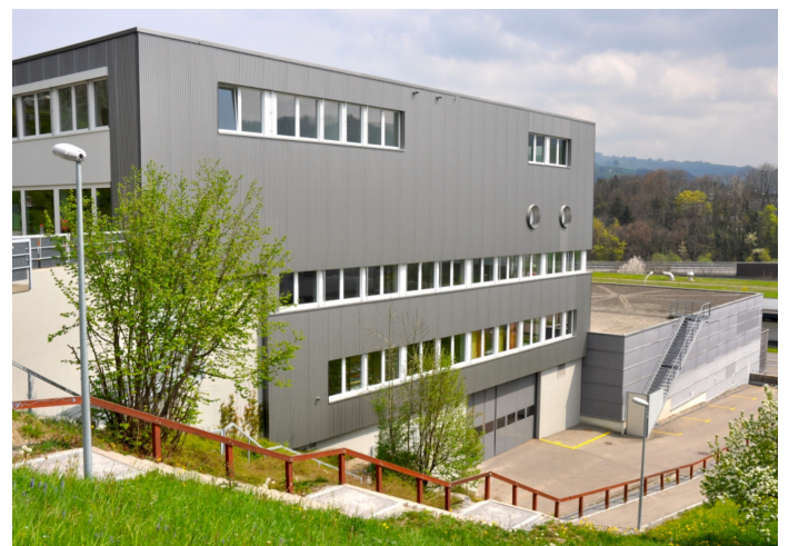
This office and commercial building in St. Gallen, built in 1981 and renovated in 2013, was equipped with a low-stroke heat pump in 2023 that provides hot water with a temperature of 26 °C. Eight geothermal probes with a depth of 280 m are used as a heat source or for cooling the building. The heat pump works with a COP of 10 and more. The heating of 100 m 2 of building area only consumes as much electricity as a 40-watt light bulb, explained Beat Wellig from the Lucerne University of Applied Sciences in a vivid comparison. Graphic: Mettiss AG
