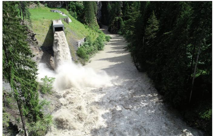
Stones, gravel, sand and fine sediments are returned to the Albula via the sediment bypass tunnel without being deposited in the Solis reservoir. View against the direction of flow of the Albula River. Photo: VAW
