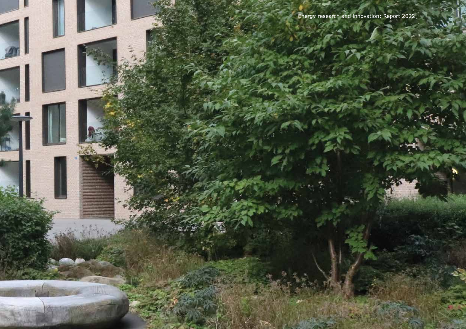
The Weltpostpark in the east of the city of Bern comprises three buildings that were built according to Minergie-Eco specifications. The development as a whole also meets the criteria of the "2000-Watt Site" label (source: B. Vogel).
