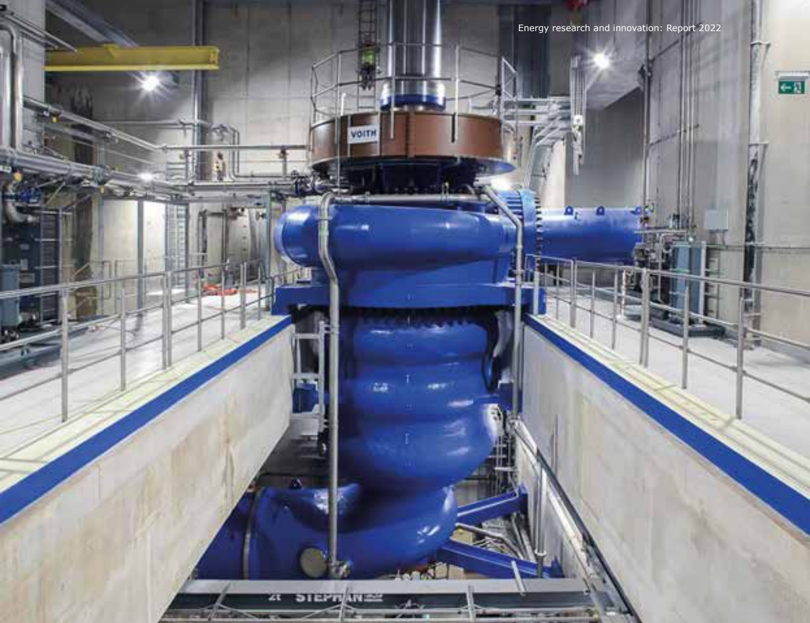
Pumped storage power plants can compensate for fluctuations in the electricity grid. To do so, they use surplus electricity to pump water back into the reservoir or bridge bottlenecks by turbinning stored water. The Veytaux power plant is now investigating how this balancing can be optimised (source: Forces Motrices Hongrin-Léman SA (FMHL)/David Picard).
