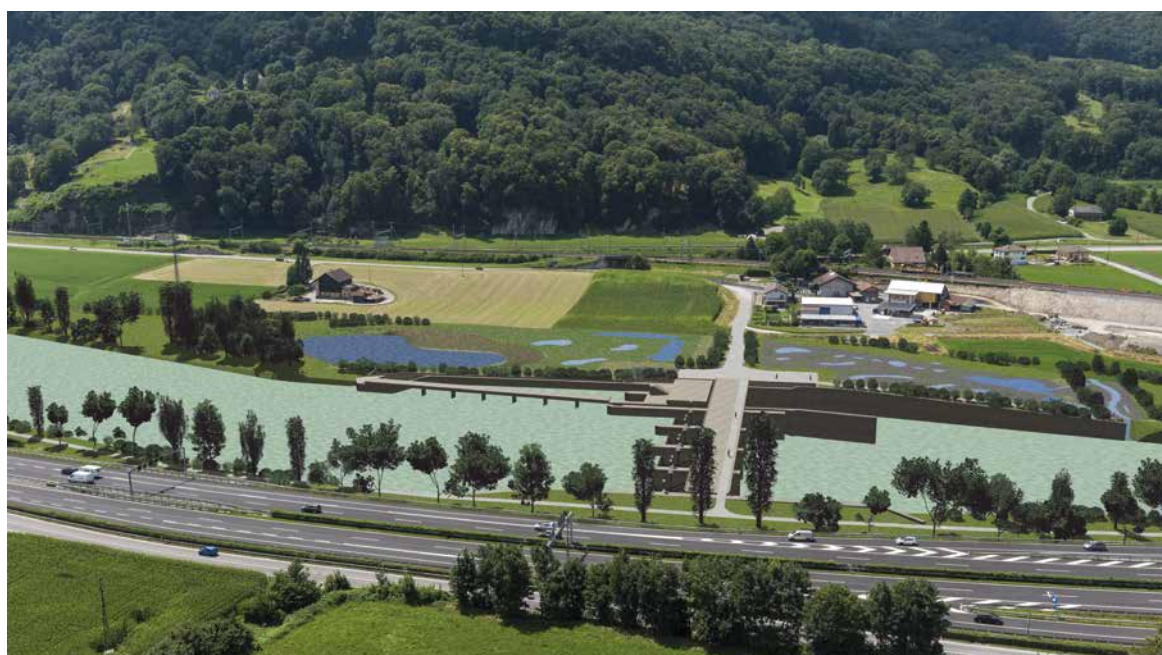
The Massongex-Bex-Rhône run-of-river power plant is scheduled to go into operation in 2028 and produce around 80 GWh of electricity annually. In order to keep the impact of the dam on the Rhone bed as low as possible, various compensatory measures are planned. To protect the fish, researchers at ETH Zurich are developing a new type of fish screen. This is intended to guide downstream migrating fish into the bypass system provided for them and around the power plant (source: MBR SA).
