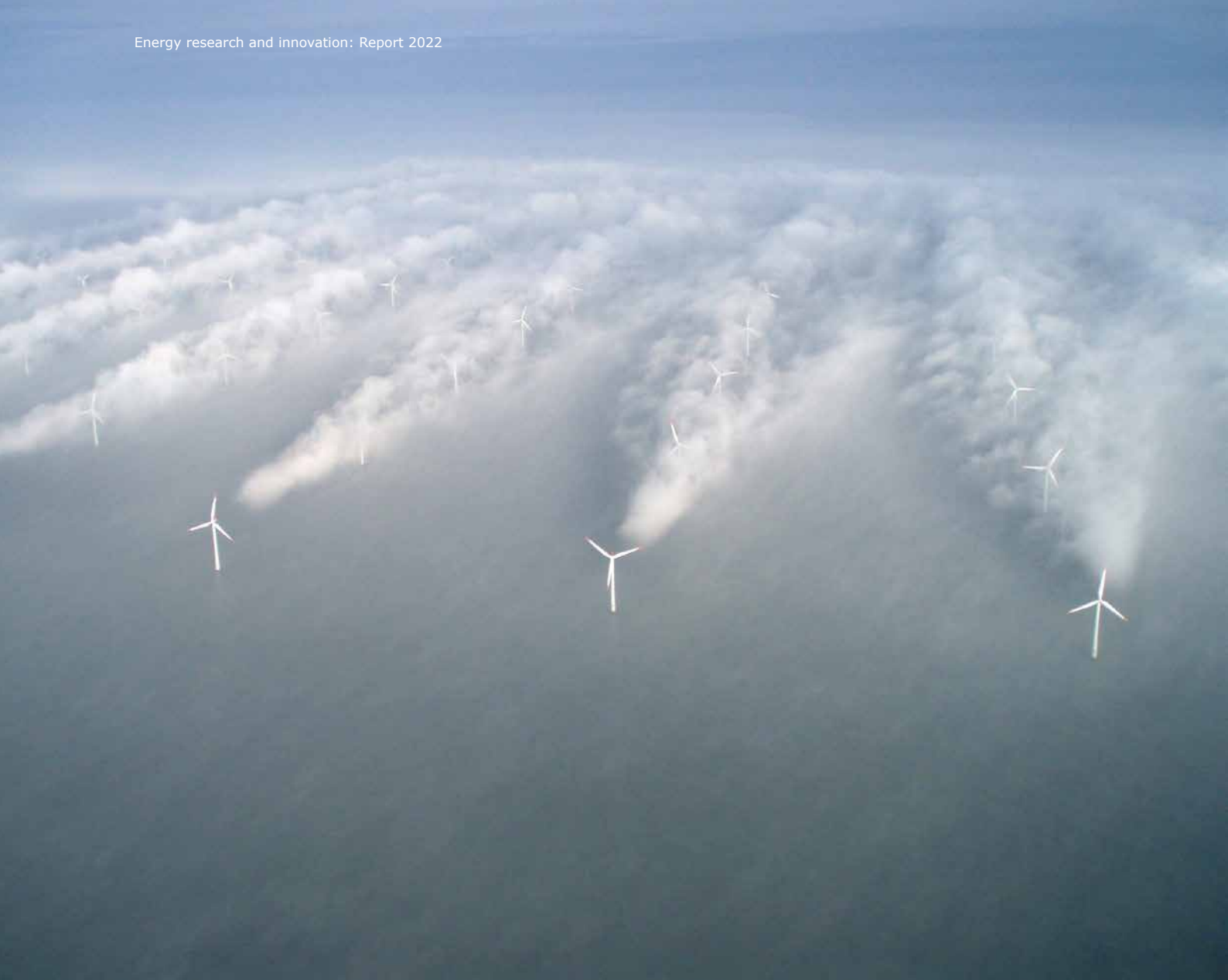
This picture of the offshore wind farm "Horns Rev 1" off the coast of Denmark shows the air circulation (wake vortices) that can occur behind a wind turbine (source: Horns Rev 1 owned by Vattenfall, photographer Christian Steiness).
