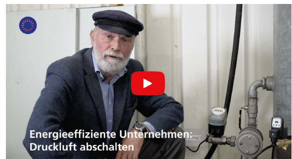
A solenoid valve automatically disconnects a machine from the compressed air network.
