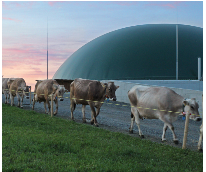
Gas from fermentation or organic matter makes it possible to produce heat and electricity from a carbon neutral energy source. Photo: Ökostrom Schweiz
