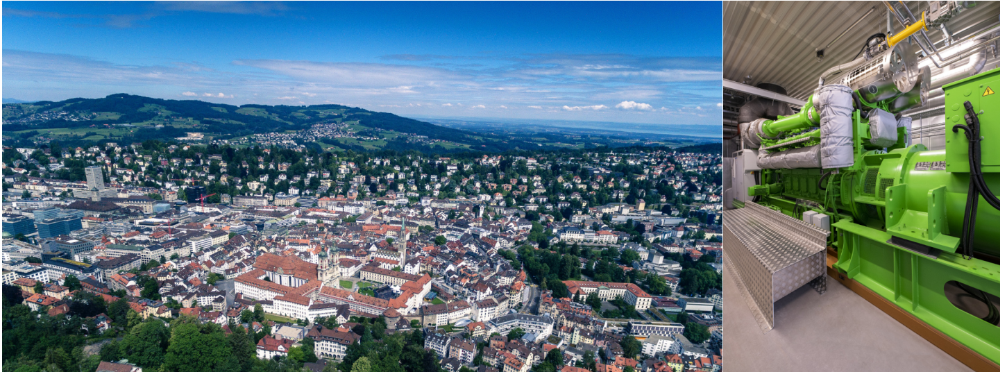
The city of St. Gallen (photo on the left) uses natural gas-fired cogeneration plants to replace oil-fired heating systems and thus reduce greenhouse gas emissions. Photo on the right: One of the two cogeneration units of the new Lukasmühle district heating plant with a capacity of 2 MW for heat and electricity production. Photo: City of St. Gallen / St. Galler Stadtwerke
