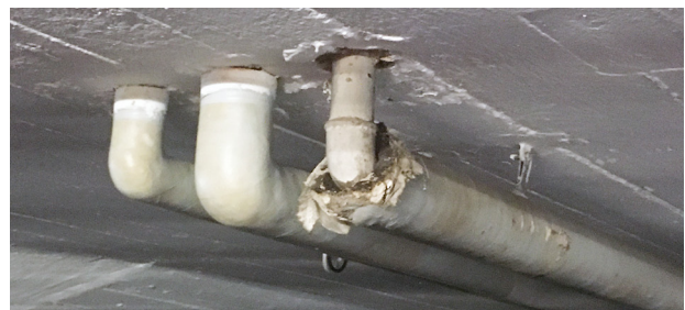
Repair defective heat insulation.
