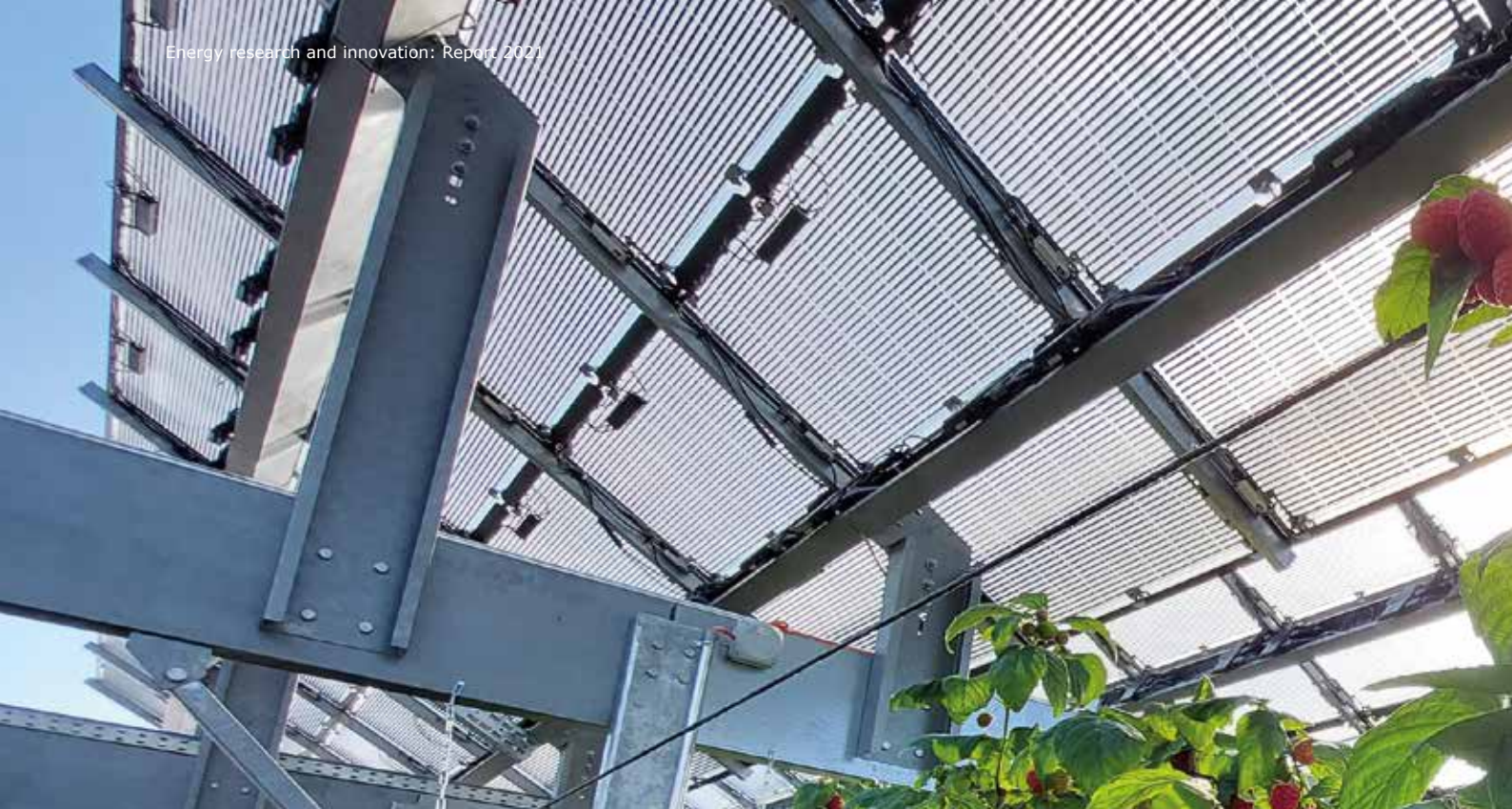
Photovoltaic pilot plant at the Agroscope research site in Conthey (VS), where modules with modifiable transparency are installed above a raspberry crop, so that the plants growing underneath are shaded to a greater or lesser extent. The solar modules were specially designed for such applications by the Swiss company Insolight (source: Agroscope).
