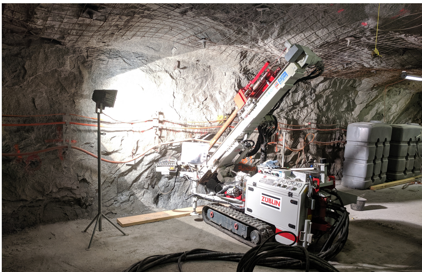
The drill rig drives a 22-cm-diameter borehole several hundred meters long into the granite of the Gotthard mountain, into which ETH Zurich scientists then insert their measuring instruments. Photo: Swiss Seismological Service at ETH Zurich, 2019
