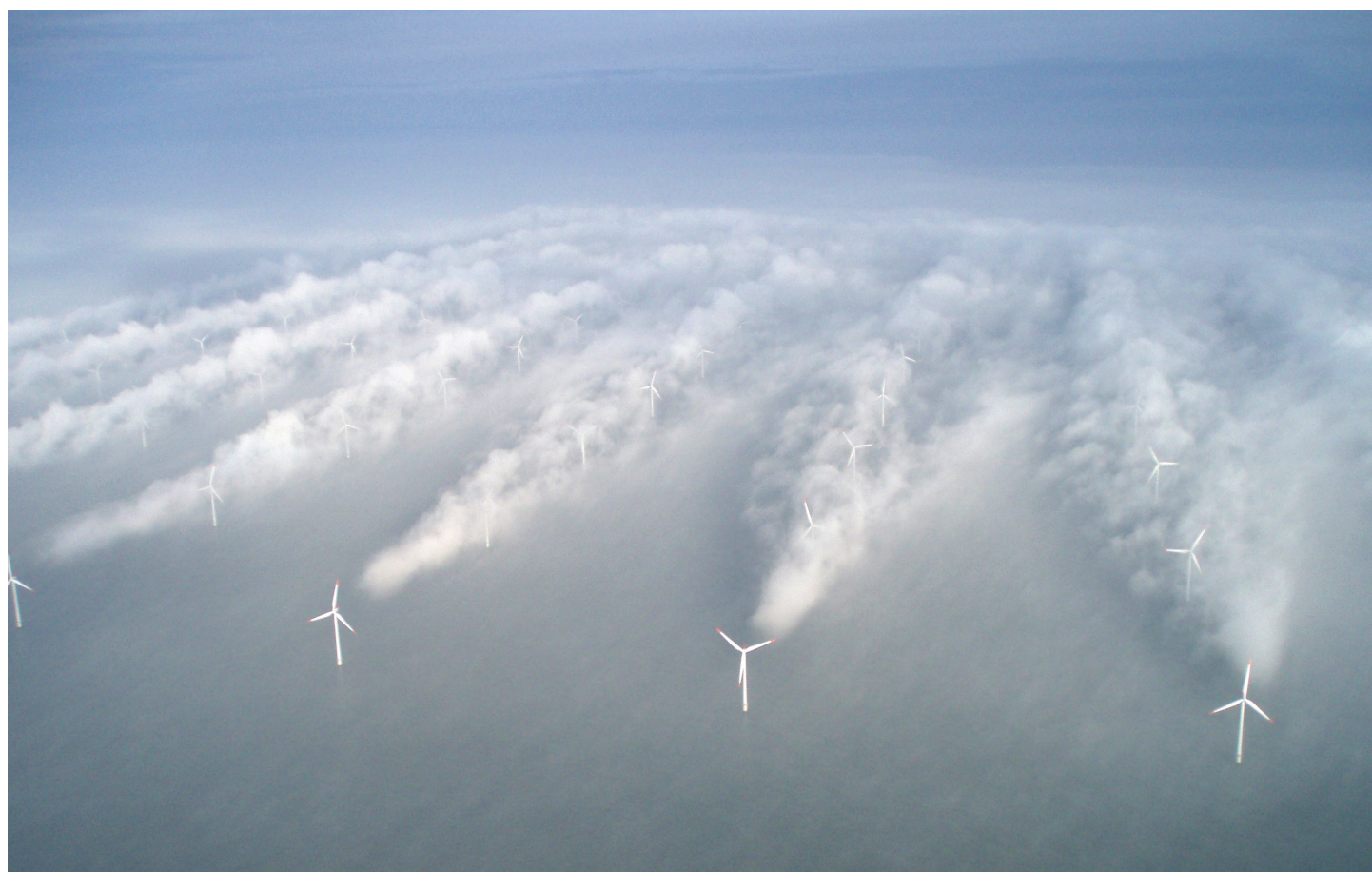
A snapshot of a special kind: Due to special weather conditions, the wake of the wind turbines in a Danish offshore wind farm becomes visible through condensation. Photo: Vattenfall/Christian Steiness
