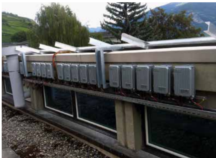
DC/DC converter for individual photovoltaic modules on the roof of the HES-SO Valais Wallis. Each of the 45 modules is connected to the DC bus via its own converter with integrated maximum power point tracker. The efficiency of the individual converters is 97 to 98 % (source: HES-SO Valais Wallis).
