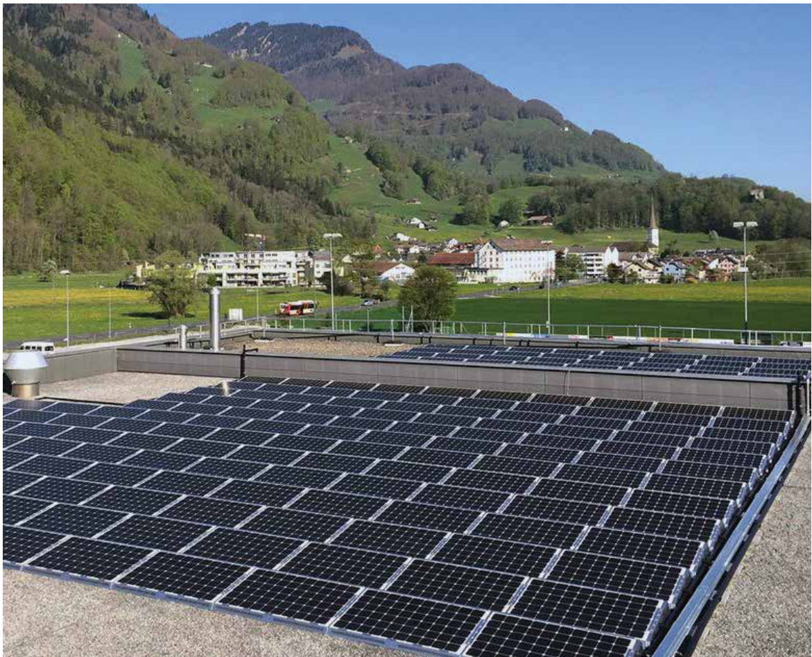
Hybrid photovoltaic thermal modules (PVT) on the roof of the linth-arena sgu (source: ZHAW).
