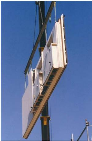
*Fig. 7: Massivholzwand
