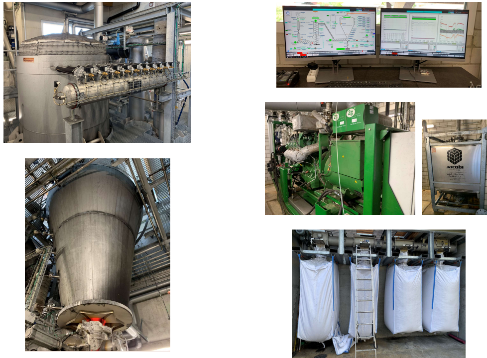
Figure 4.18: Synkraft plant in operation in Switzerland. Left: Floating bed reactor, right: Engine, filter detail, biochar. Photos: T. Nussbaumer, 2024.
