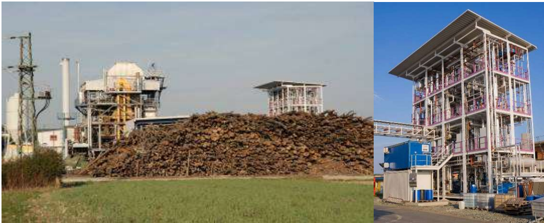
Figure 5.9: Process development unit TRL 7, operated within the European Union project BioSNG in 2008/2009 [4.6].
