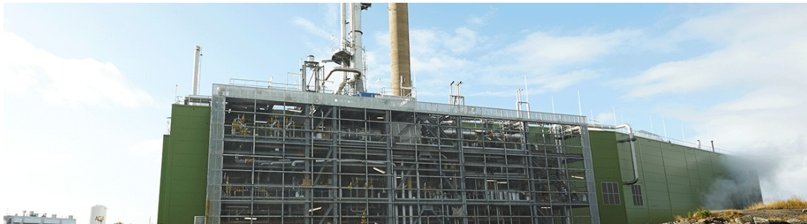
Figure 5.7: Gothenburg BioGas plant in Sweden, commissioned 2014 [4.10].
