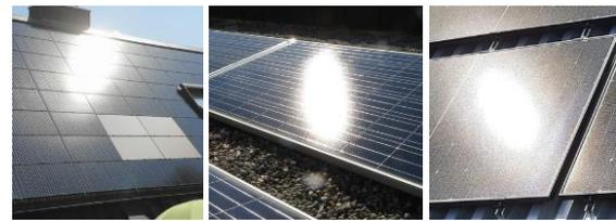
**Figure 4:** The appearance of glare is usually elliptical.
