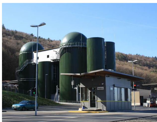
Biogasanlage KBA Hard, Beringen (SH)
